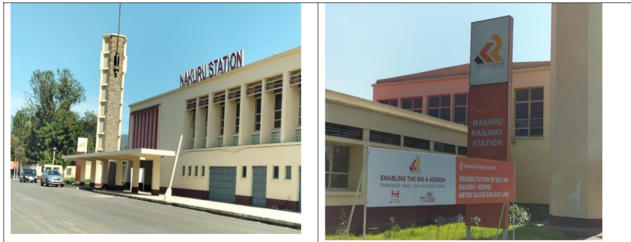
Picture 2: Images of Nakuru Railway Station (under renovation & revamping)
