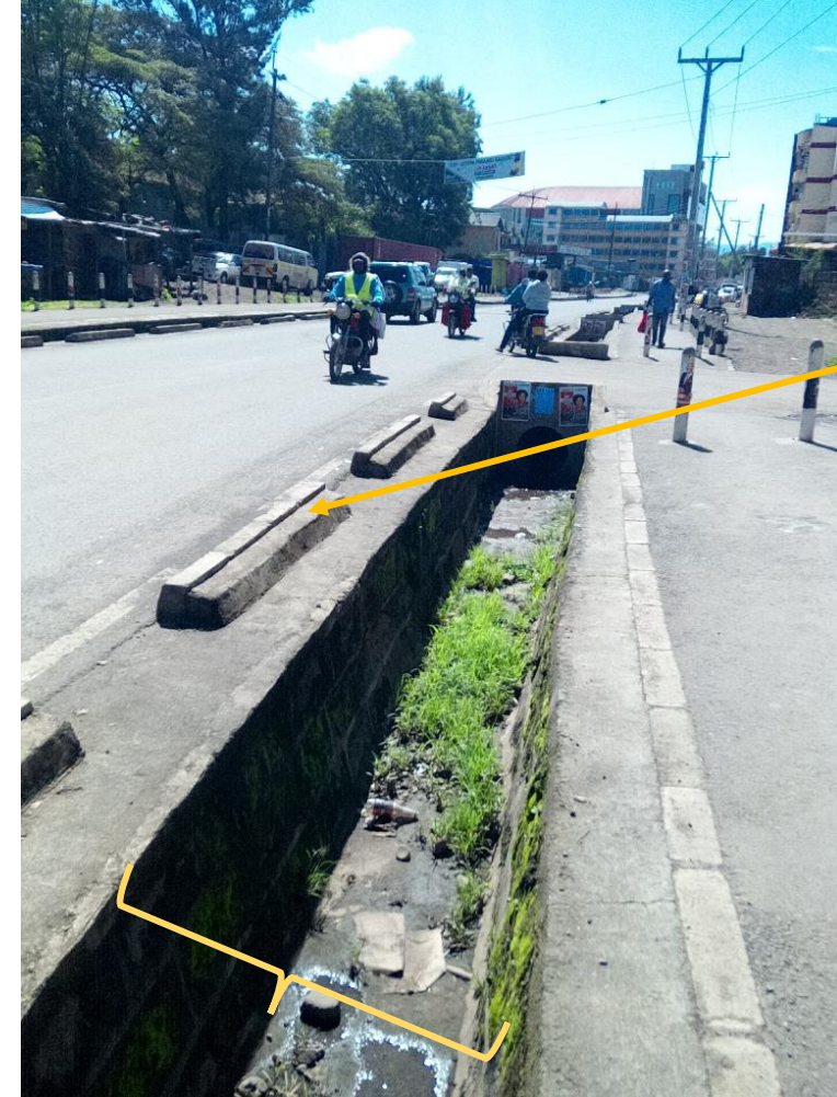
Open Storm water drains
