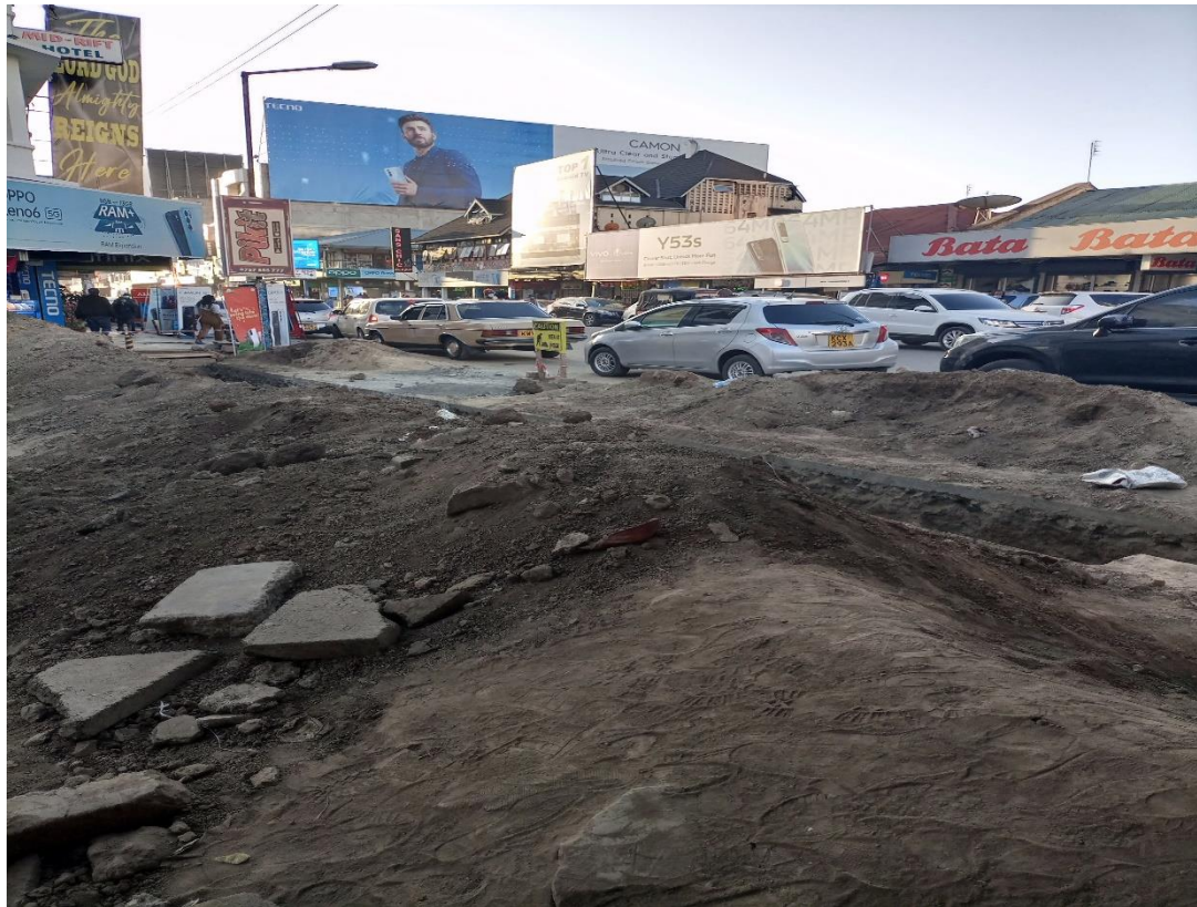
Sidewalk Construction on Kenyatta Avenue
