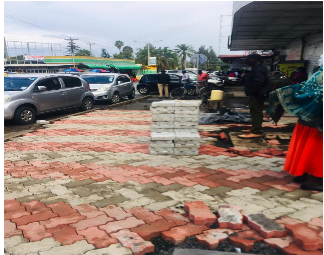
Sidewalk Repair on Kenyatta Avenue
